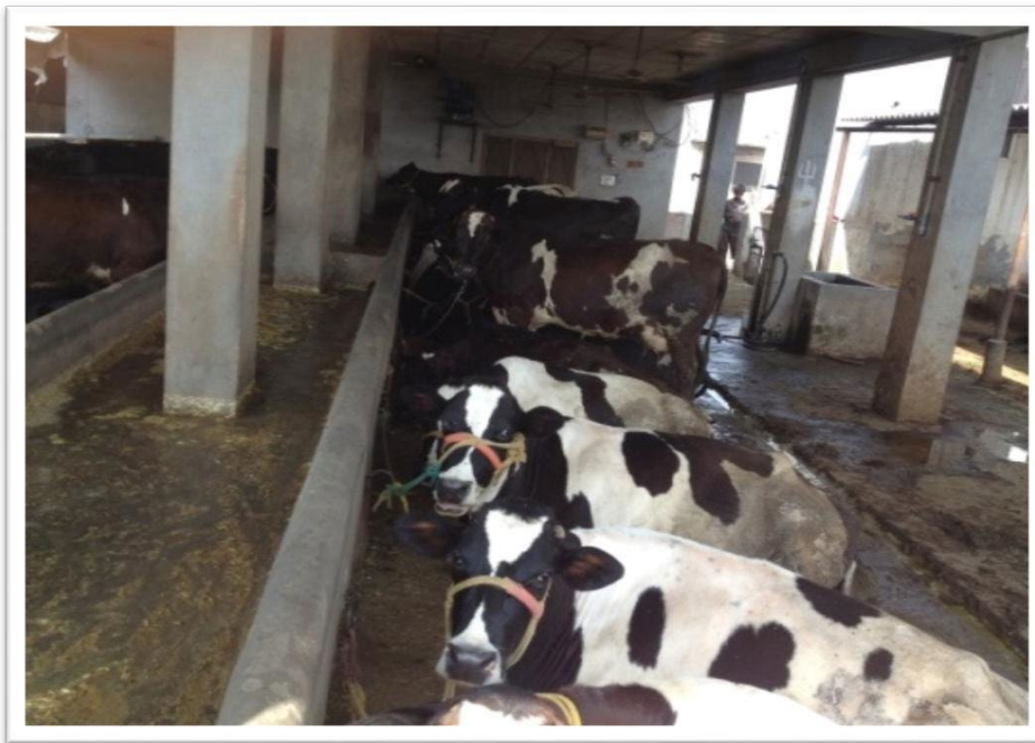
Figure S3 Tie-house with inadequate height and concrete flooring at a small farm.
